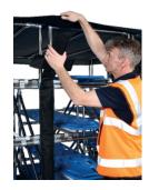
Attach the two Velcro door pillars to the racks. Ensure you get it the right way up.
